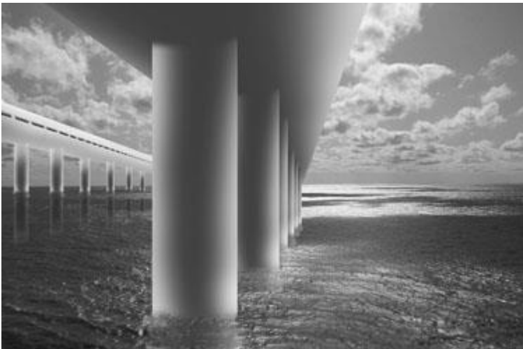
The twin spans of the Bering Strait Bridge. The original span (closest) is the Charles Alton Ellis Memorial Bridge . The second span is the Joseph Baermann Strauss Memorial Bridge .
