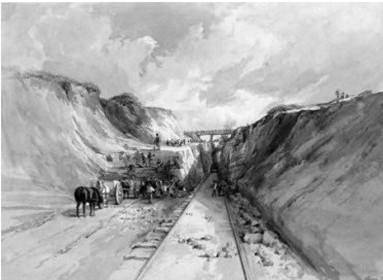
Building the Great Western Railway.
