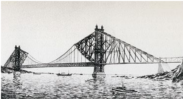
Joseph Strauss' original design for the Golden Gate Bridge.
