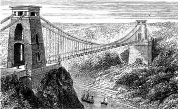
Brunel's Clifton Suspension Bridge became the symbol of the City of Bristol.
