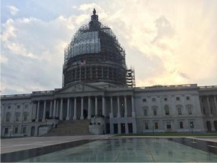
Capitol Dome in Scaffolding. Photo by R. S. Kirchman
