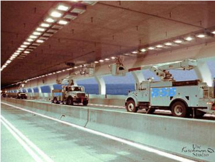
Maintenance operations on the Bering Strait Bridge. Graphic by Bob Kirchner
